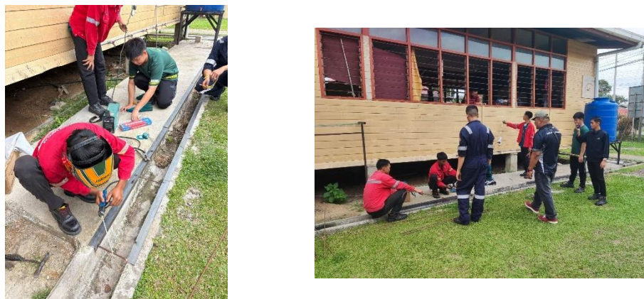
Figure 11. Fitting the Grates into the Edges of the Drains
