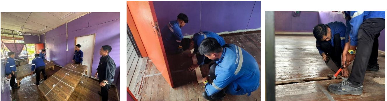
Figure 7. Volunteers Replacing Planks on Wooden Floor
